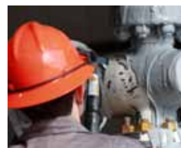
11"-5K Wellhead 3 hours coating application
